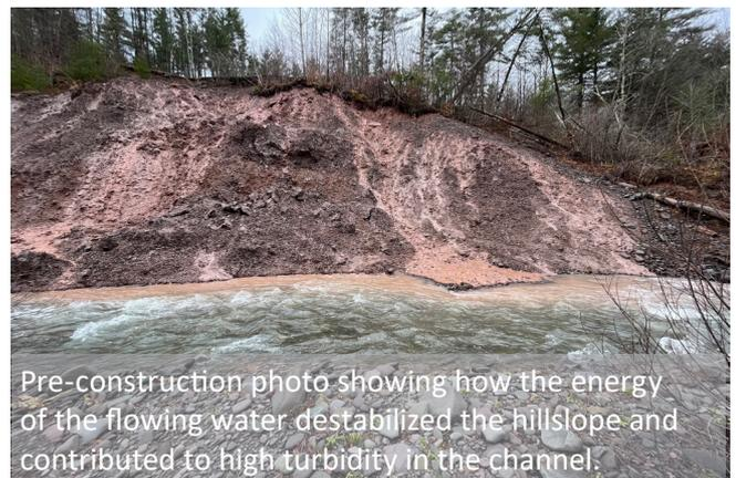
Pre-construction photo showing how the energy of the flowing water destabilized the hillslope and contributed to high turbidity in the channel.
