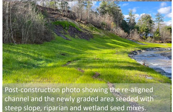
Post-construction photo showing the re-aligned channel and the newly graded area seeded with steep slope, riparian and wetland seed mixes.
