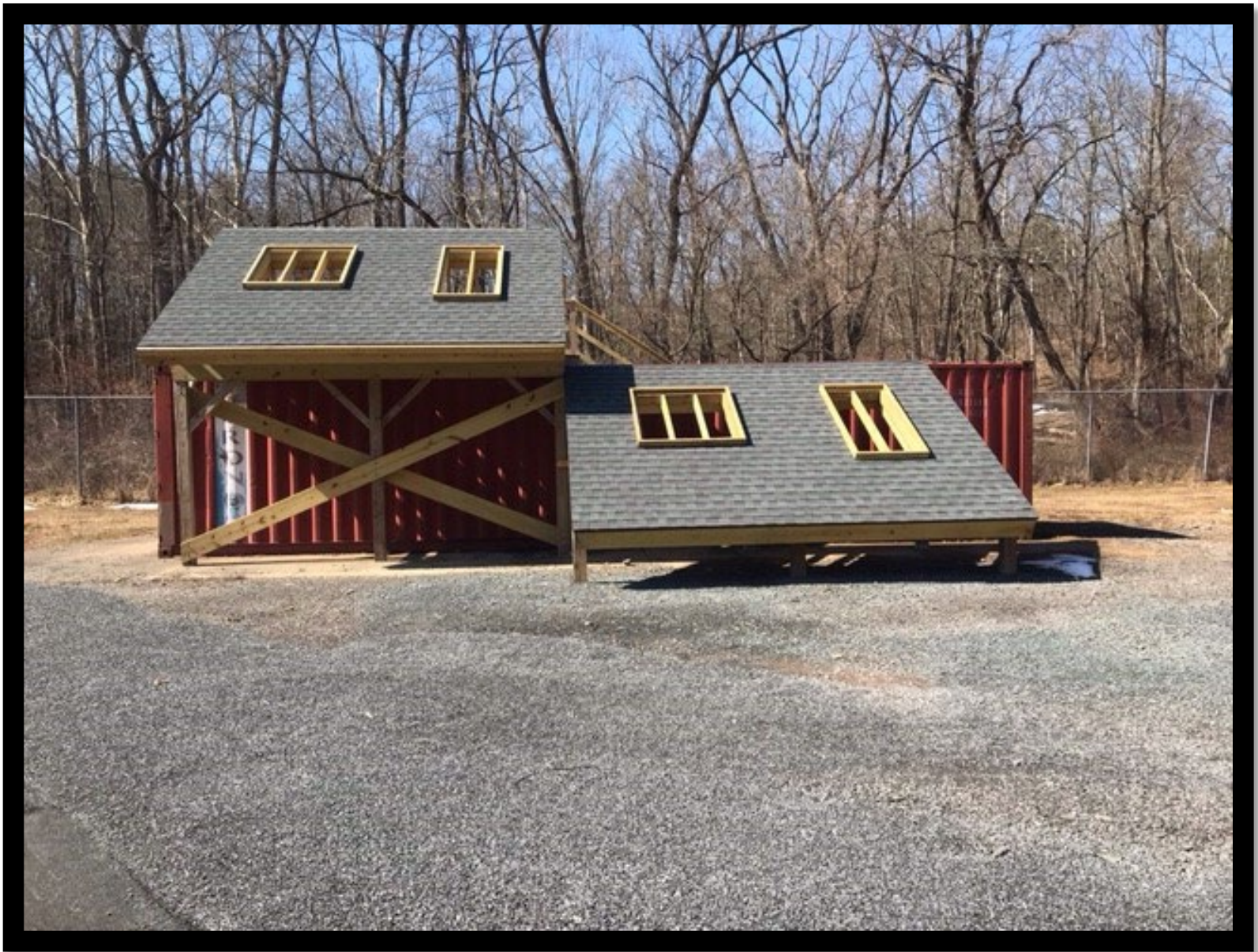
Greene County Buildings and Grounds Staff were able to finish constructing a stationary ventilation training prop for fire training. This roof simulation prop gives fire departments the ability to conduct realistic training scenarios and simulations of cutting ventilation holes in a controlled environment.
