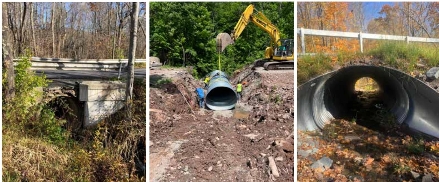
*Downstream (north) view of pre-, during, and post-construction (left to right) of the culvert replacement project.*
