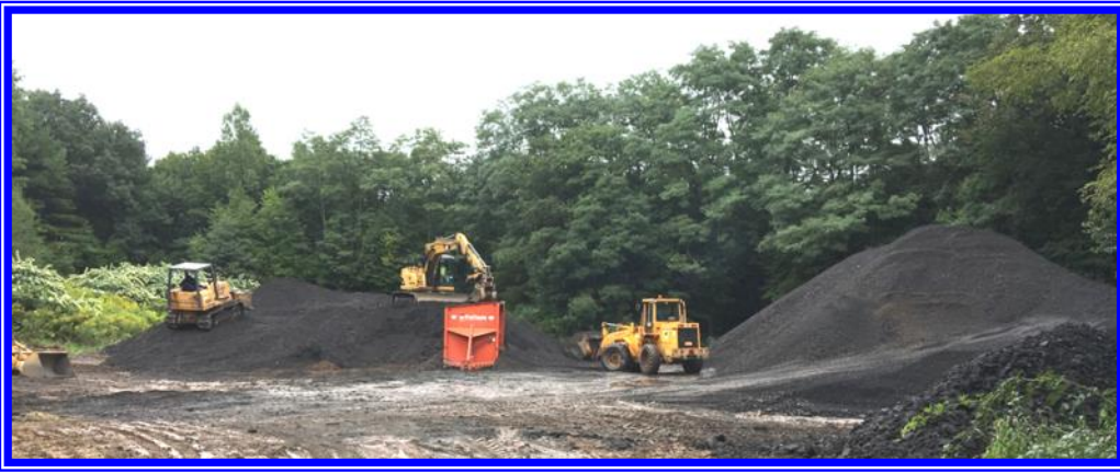
Crushing & Stockpiling the recycled asphalt millings located at the County Farm, in the Town of Cairo.
