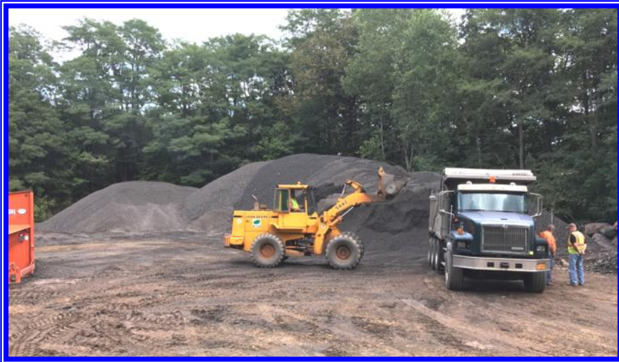
Crushing & Stockpiling the recycled asphalt millings located at the County Farm, in the Town of Cairo.
