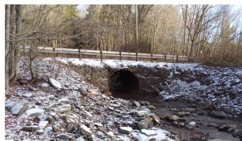
The original County Route 78 steel pipe culvert.
