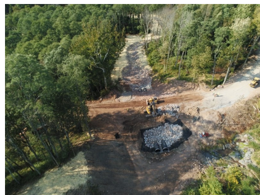
Aerial photo taken during construction of the access road and dewatering channel that were included in Phase 1 of the Batavia Kill Full Channel Stream Restoration Project at Red Falls.
