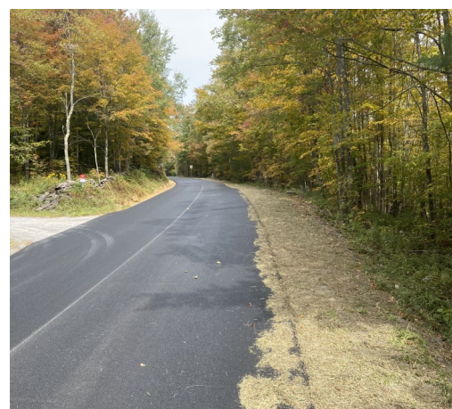
GCSWCD staff applied seed and mulch after the local highway department did shoulder work along County Road 3 in Halcott.
