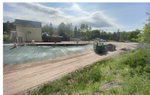
GCSWCD staff using a hydroseeder at the Windham Transfer Station after a scale replacement project.
