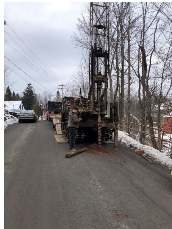
Geotech drilling, Railroad Avenue
