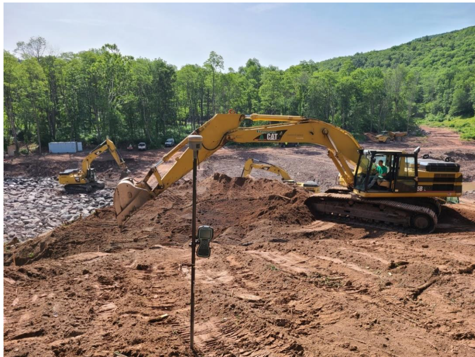
Batavia Kill Full Channel Stream Restoration Project at Red Falls Contract 2 Phase 1 bank grading and riffle installation.
