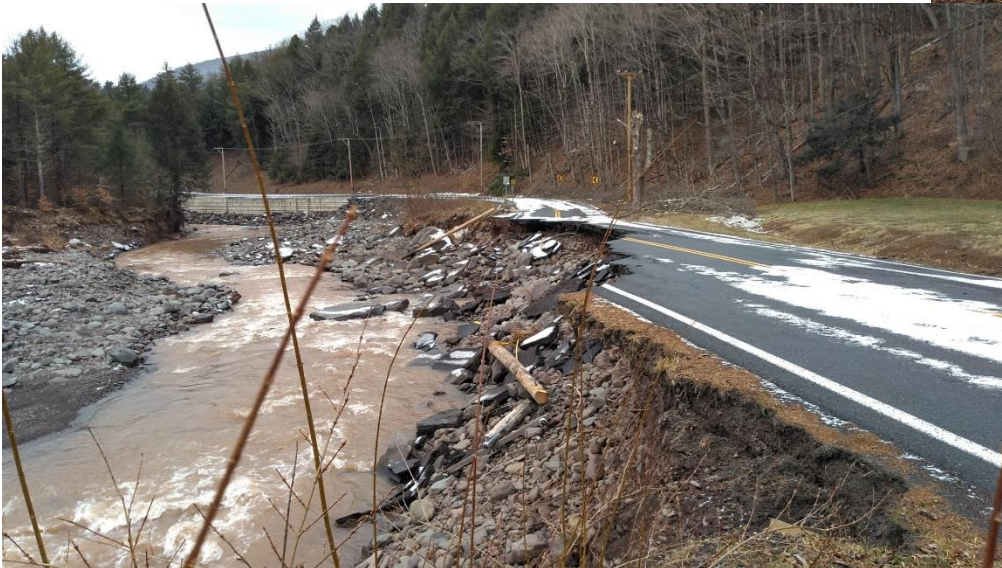
Before and after photos of County Route 17 Embankment Stabilization
