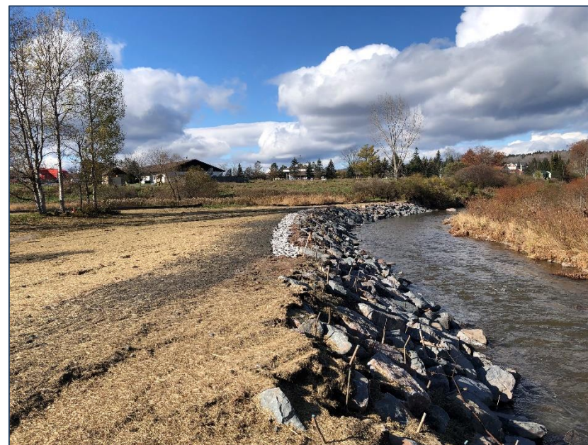
Streambank stabilization along the Batavia Kill.
