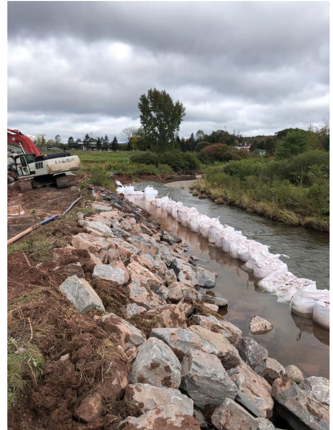
Revetment installation and sand bag cofferdam
